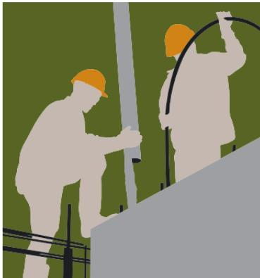
In addition, vibrators should never be used to move concrete horizontally within the formwork because this can lead to aggregate segregation, removal of form release agent, and unnecessary abrasion/scouring of the panel overlay surface. Instead, lower the vibrator vertically into the concrete at regularly spaced intervals and allow it to descend by gravity. Hold the vibrator stationary until adequate consolidation is attained (approximately 5-15 seconds), and then slowly withdraw it<sup>3</sup>.
