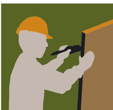
be sure to reseal any cut edges. This will slow the migration of moisture and alkalis into the panel edges. Without resealing, cut edges will break down faster, become weaker, and require replacement sooner.
