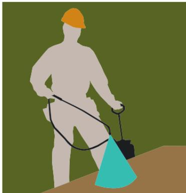
In any event, the type of release agent used should correspond to the type of finished surface or appearance required. For example, release agents with waxes or silicone should not be used when the concrete is to be painted.
